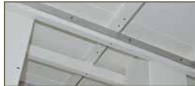
Aluminum support framing underneath all table tops
